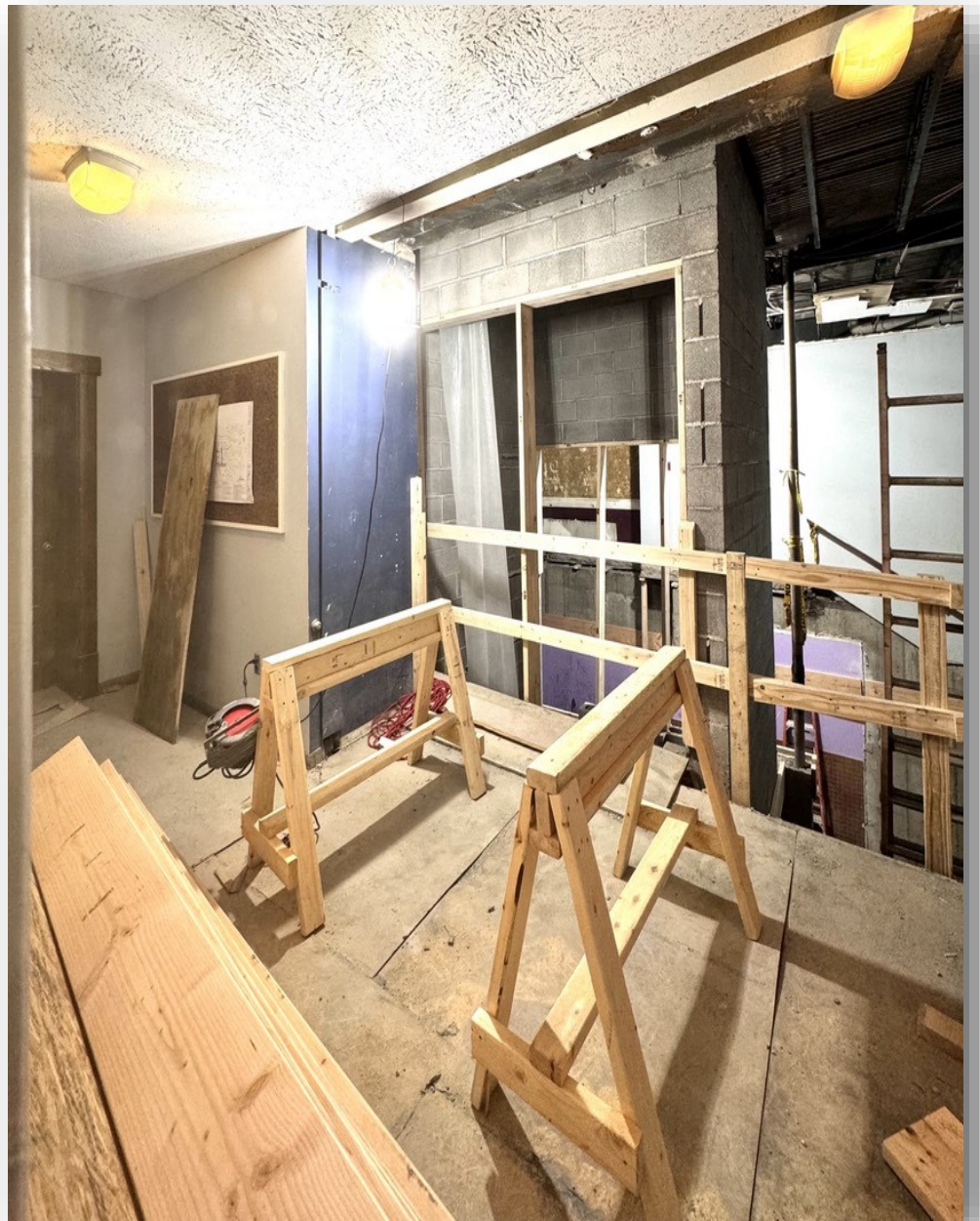
The lobby and elevator shaft as of July 2
