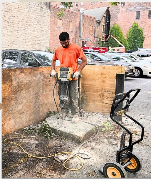
Jackhammering out the cement pad in the parking lot
